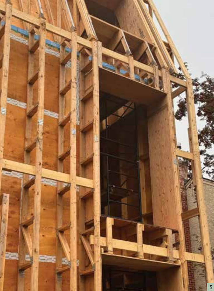
5. Wood floor trusses used in the wall construction are fully thermally isolated from the foundation to prevent heat loss to grade.
