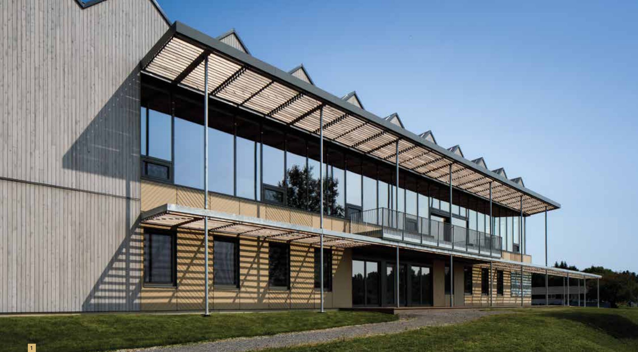
1. The double south-facing brise soleil cuts solar radiation in summer while maximizing solar gain in winter.
